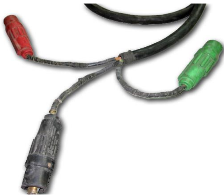
Unsafe Splay with exposed conductors
