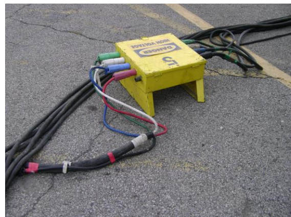
Misapplication of multi-conductor used with single-conductor Cam Lok connectors.
